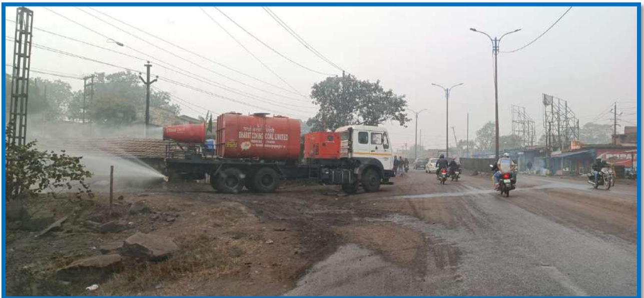
Picture 2 – Water Sprinkling on Transportation Road
