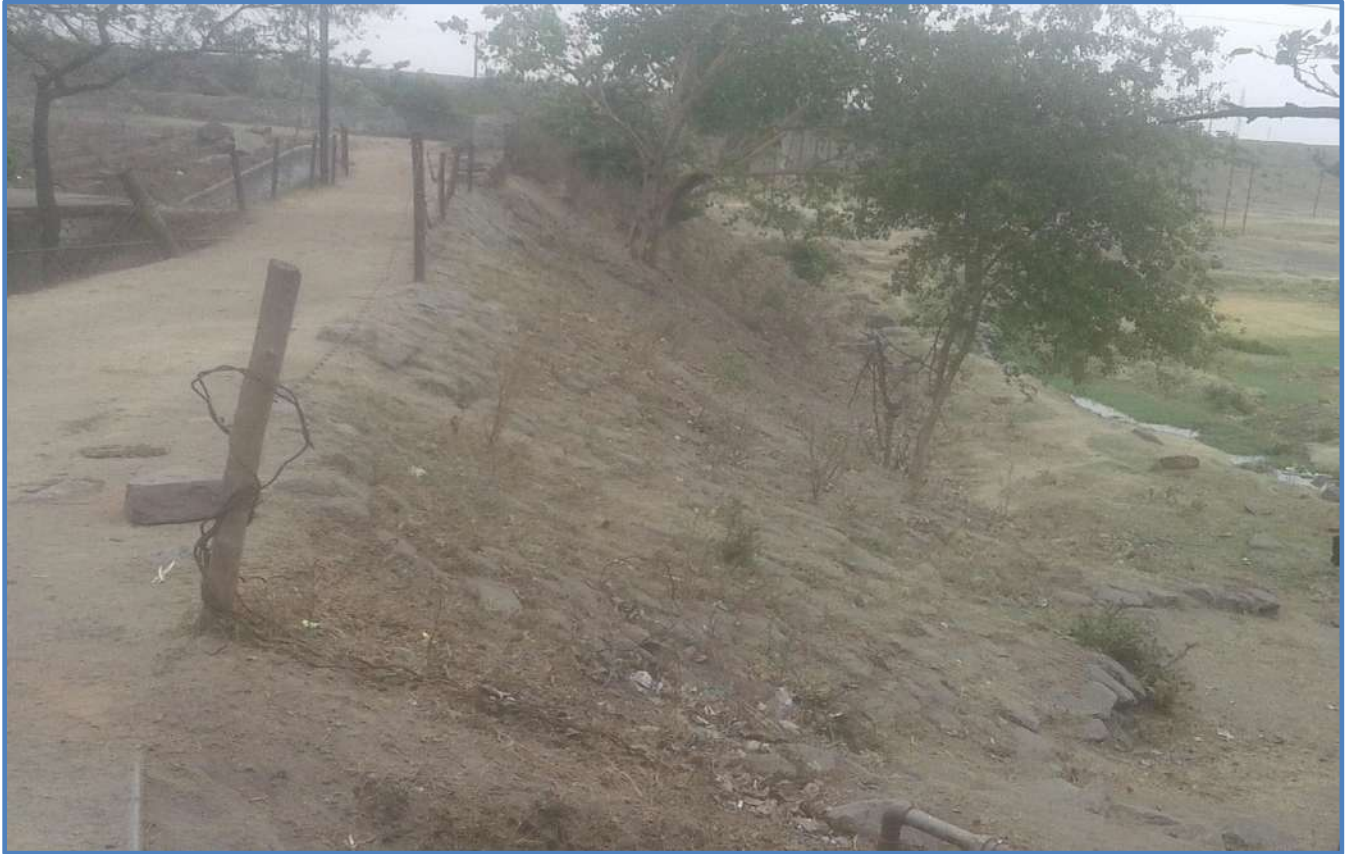
Picture 3 - Stone Pitching/embankment at Kari Jore
